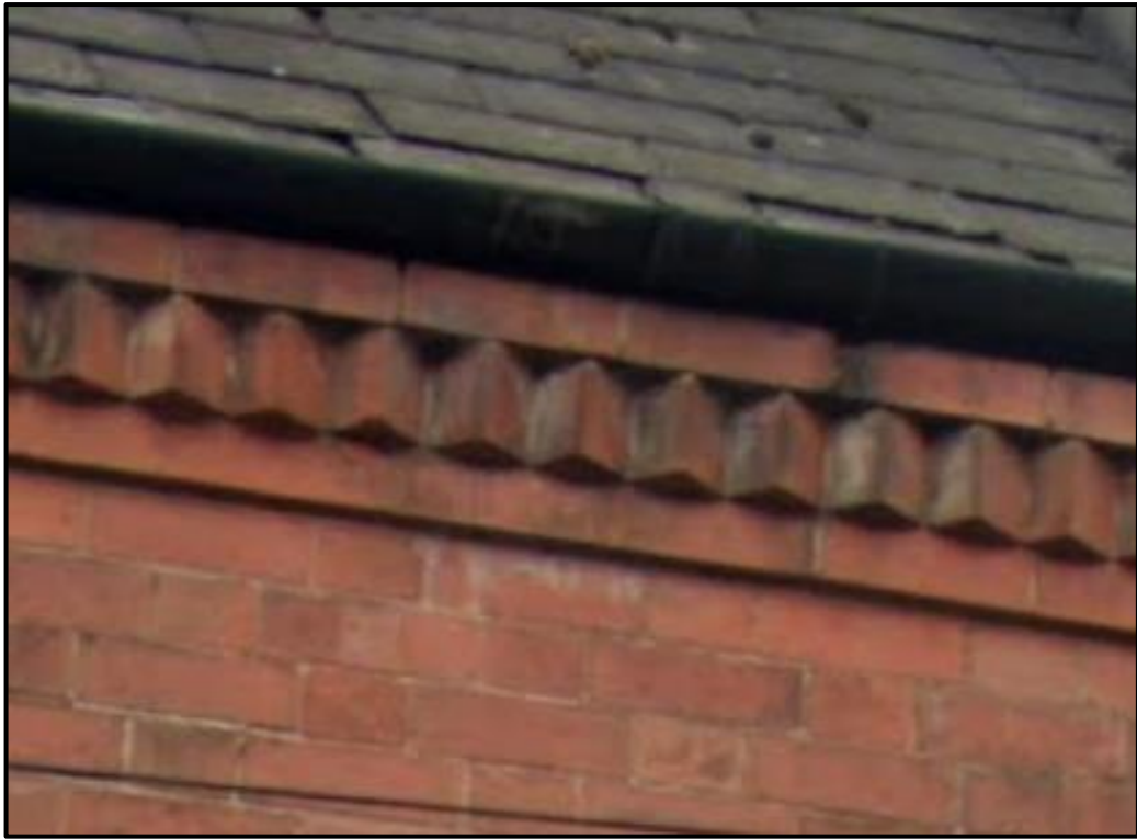
Photo: Dog Tooth Eaves or Cogging
